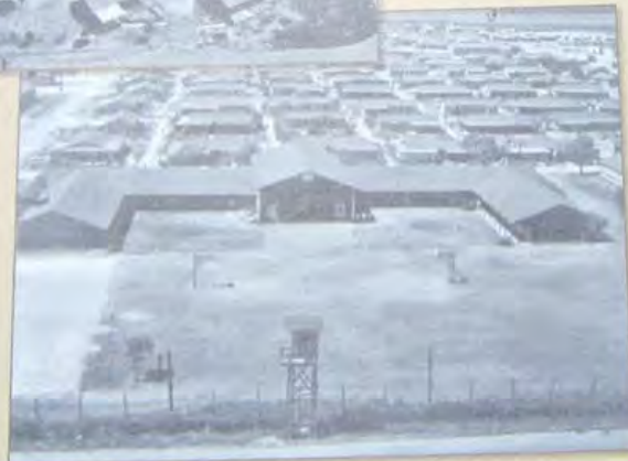
Aerial view of Federal High School (looking north), courtesy of Carroll Brincefield.
